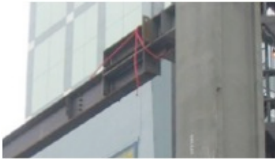
Figure 3: 'Dog-leg' beam connection
